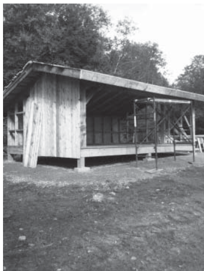
Phil's shelter in progress.
